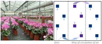
Climate management software for greenhouses enables air mixing and heating to be controlled and combined with precision, switching them on and combining them only when necessary.
